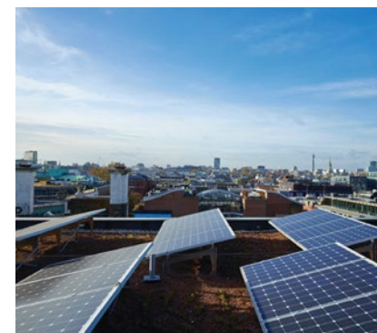
Integrated on-site energy production and biodiverse roofs
