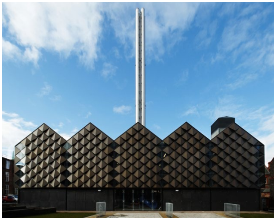
Heating Infrastructure Energy Centre, University of Liverpool
